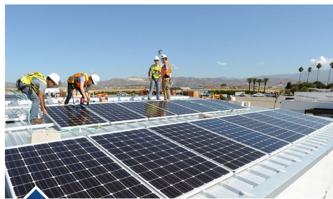
Solar panels being installed in California.
