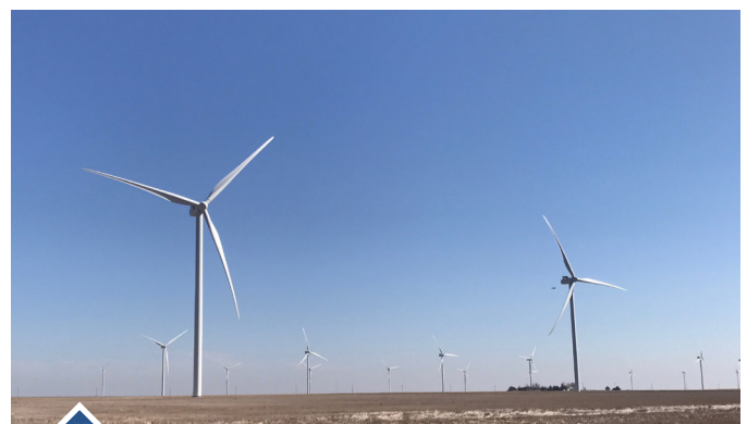
Wind turbines in Kansas.
