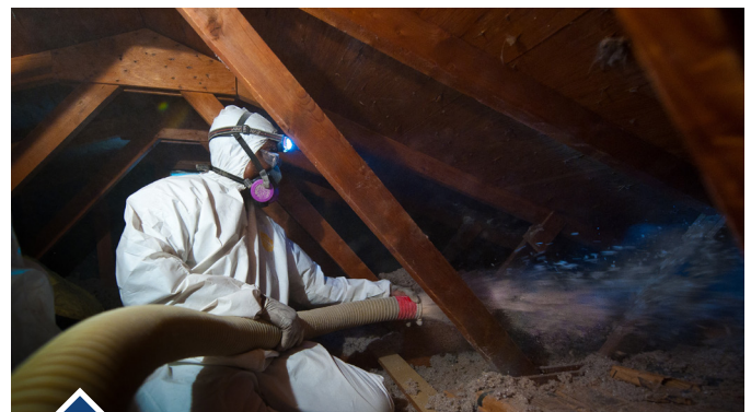
Home weatherization saves energy and money.
